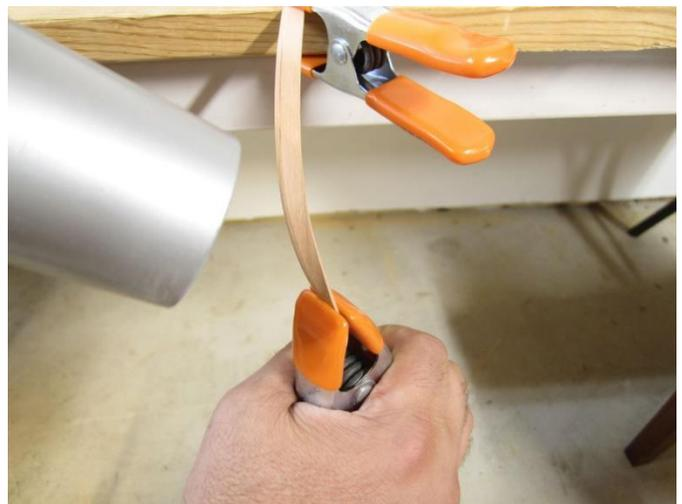
The photo above shows how I form the planks. I use a hair dryer on its hottest setting. Clamp the plank
